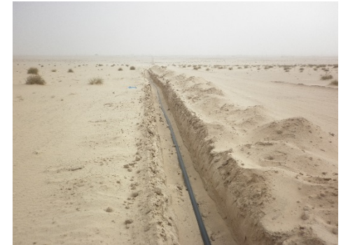
Trenching/Fiber Laying
